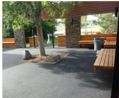
Patio project with pour-in-place surfacing Edmonton, AB
